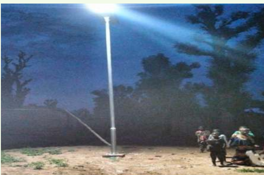
Solar Powered Street Light
